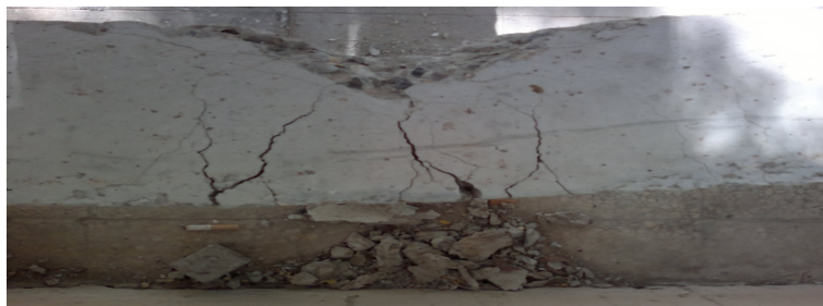
Fig. 4: Failure of control Beam in Compression with wide Flexure cracks
