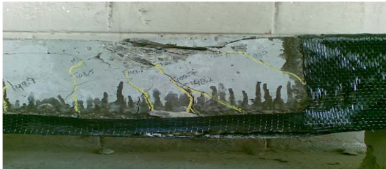
Fig. 6: Diagonal shear compression failure
