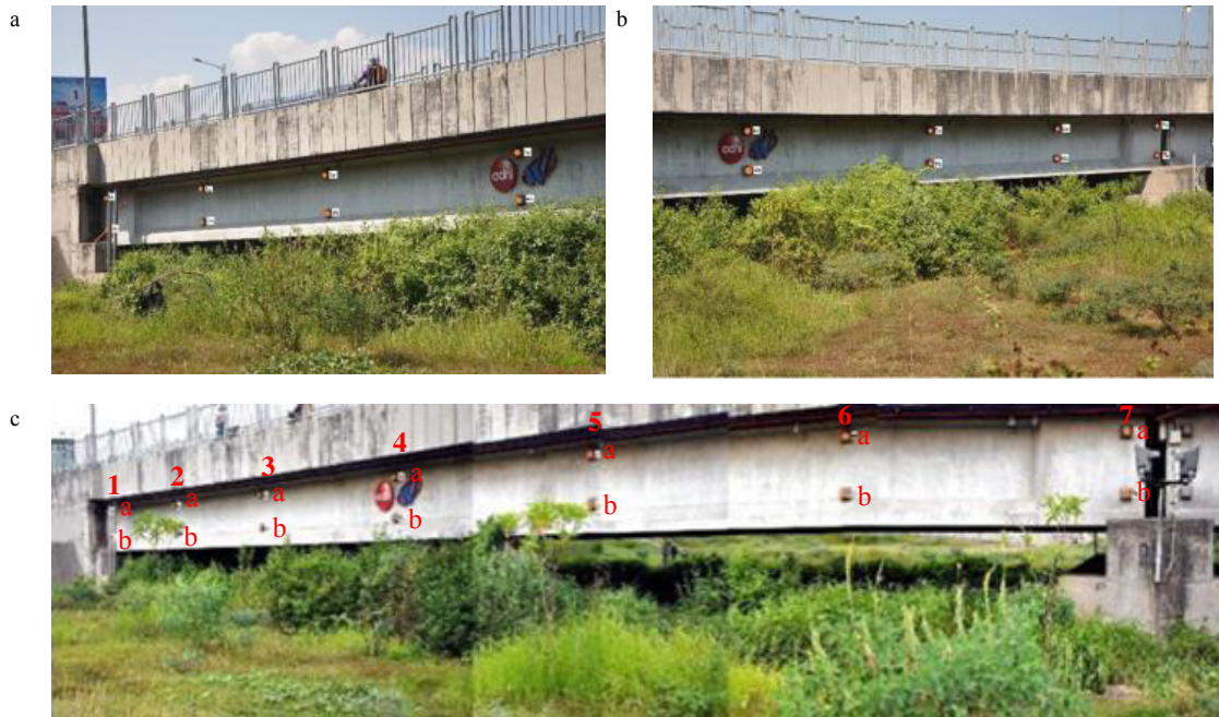
Fig.5. Captured images overlapping one another of bridge spans in Madura side with distribution of GCPs (a). First image; (b). Second image (c). mosaicking of the first and second image.
