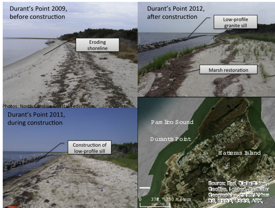
Fig. 5. Durant's Point Living Shoreline, Dare County, N.C. Durant's Point is a privately-owned property located on a peninsula at the entrance to Hatteras Harbor in Pamlico Sound on the Outer Banks of North Carolina. The living shoreline consists of 320-foot long low-profile granite sill with restored marsh. Top left: eroding shoreline, bottom left: construction of low-profile granite sill, top right: marsh restoration, bottom right: map of Hatteras with Durant's Point labeled.
