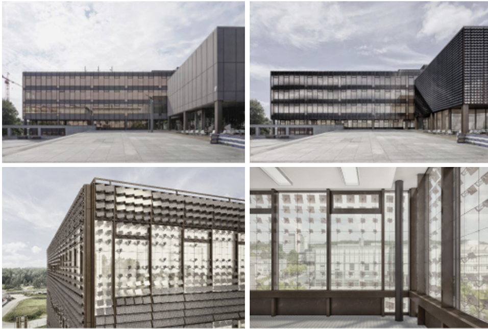
Fig. 4 The Adaptive Solar Facade as a retrofit measure on the HIL building of ETH Zürich. Top left: Photograph of the building. Top right: Photomontage of the building with the ASF. Bottom left: Close-up view. Bottom right: View from the inside. (Images by Christian Studerus.)
