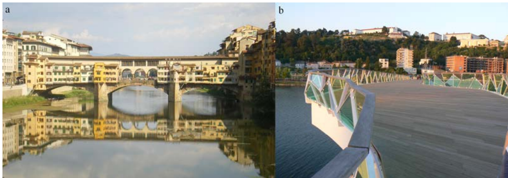
Fig. 3. (a) Ponte Vecchio in Florence; (b) Pedro and Ines footbridge in Coimbra.
