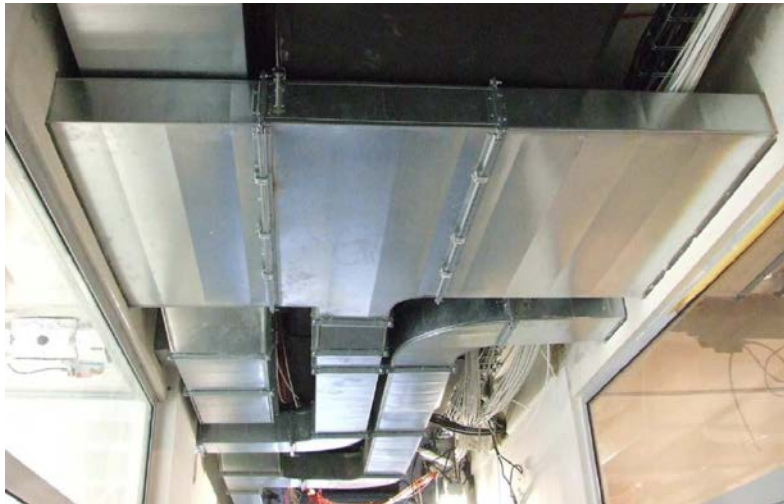
Figure 3 Complicated installation work (ceiling in corridor area, not finished)
