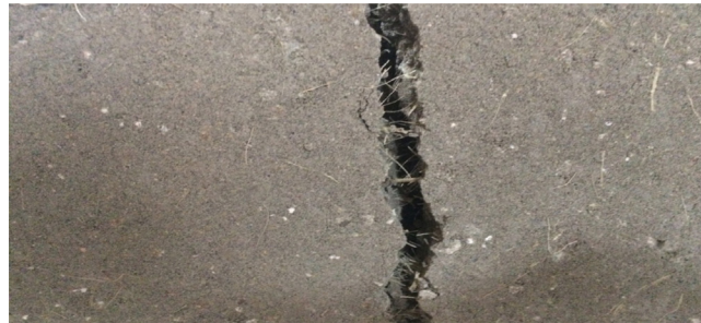
Fig. 8. Banana Fibers Bridging the B-CEB Cracks During Failure.
