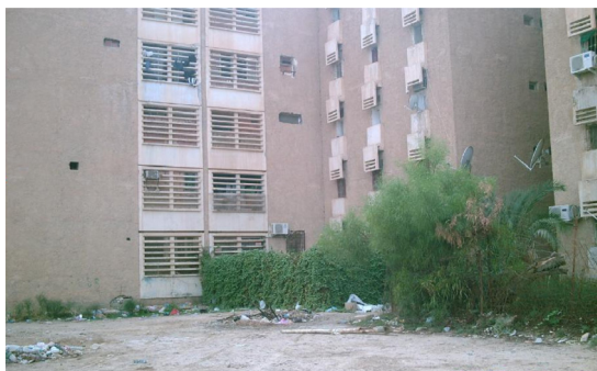
Photo 2 Gardens organized poorly and improperly kept.
