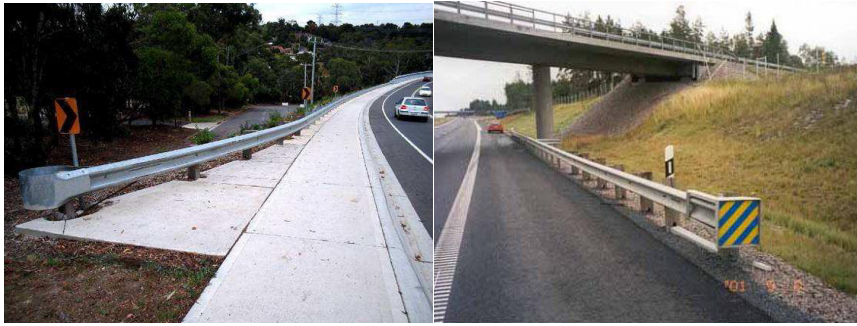
Fig. 3. Crashworthy barrier terminals ([5], left & [1] right)
