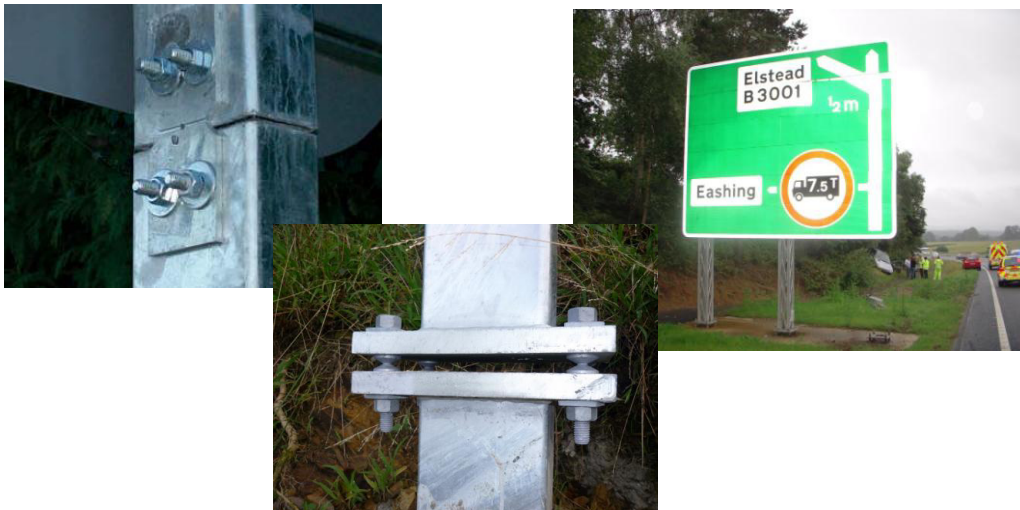
Fig. 7: Passively safe support structures [2]
