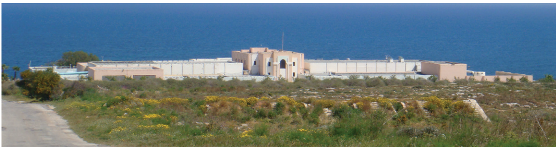
Fig. 2. Pembroke RO plant; (photo by the author)
