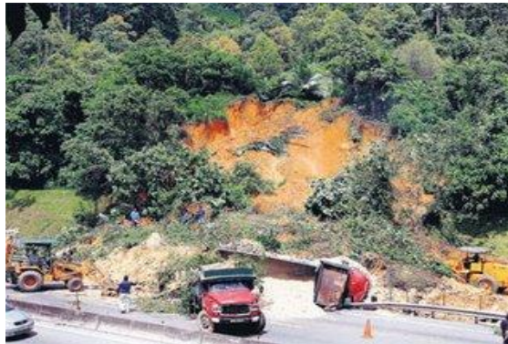
Figure 1: Landslide at North-South Highway near to Kuala Kangsar, Perak [9]
