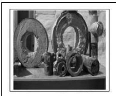
Figure 5. Scaling of pipes
