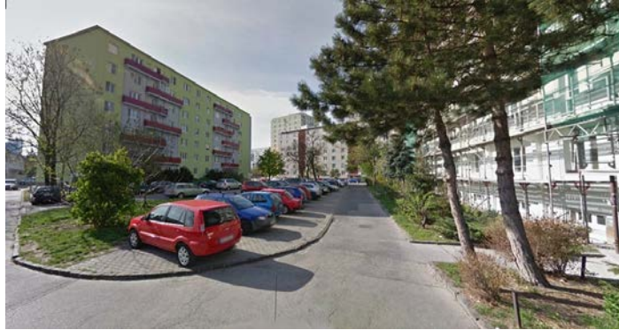
Fig. 3. The former green spaces equipped which children playgrounds are transformed to parking places – example from housing estate Hostinského. Source: Google street view.
