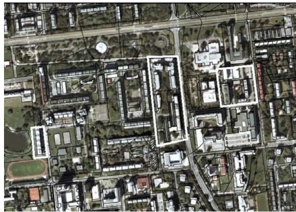
Fig. 1. Losses of open green spaces by densification of urban structure by housing, commercial, and civic amenities development, example of housing estate Ružinov, Source: https://www.geoportal.sk/sk/aplikacie/mapka/ .
