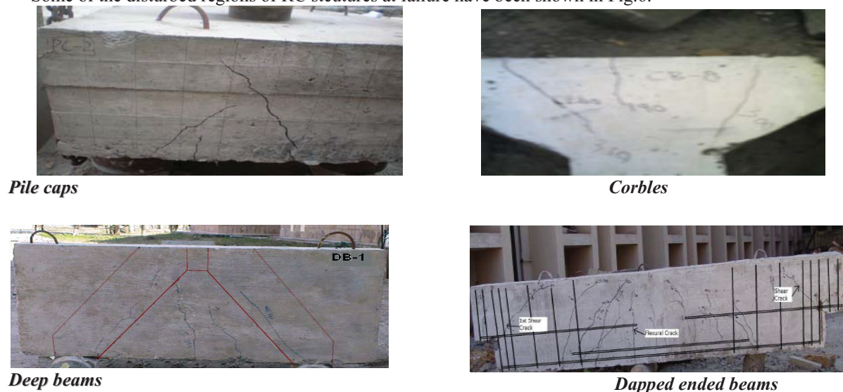
Fig.6 Typical failure modes of deep pile caps, corbelsl, deep beams and dapped ended beams.
