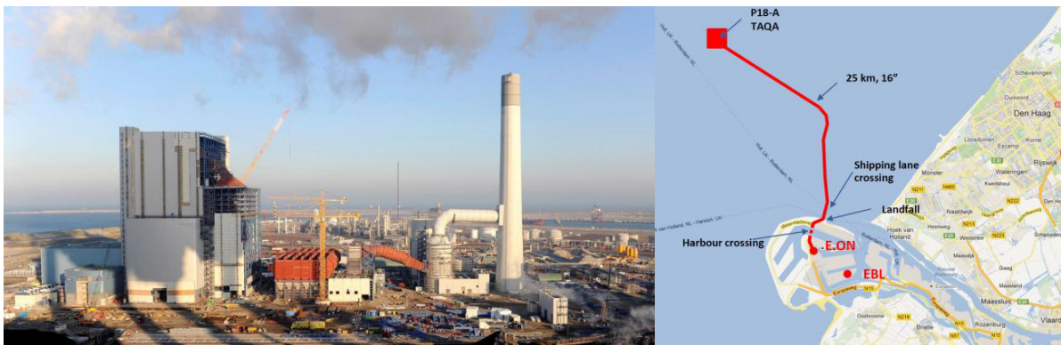
Figure 5: Left: The capture-ready Maasvlakte Power Plant 3 under construction (ROAD project). Output 1.070 MW e (without CCS), efficiency 46% (LHV). Hot commissioning started in 2013 with planned commercial operations in 2014. Right: Location of the ROAD project and its CO 2 transport lane at reclaimed land at the Rotterdam harbour. Pipeline characteristics: 5 km onshore, 20 km offshore. Diameter: 400 mm nominal diameter (16 inch) insulated steel pipe, transport capacity: 5 Mtpa (dense). Maximum design specifications: 140 barg, 80°C.
