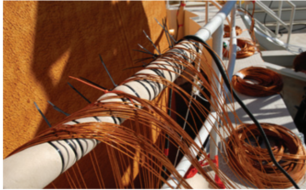
Fig. 7. Instrumentation wiring for testing the structural integrity of the space shuttle Discovery's external tank.
