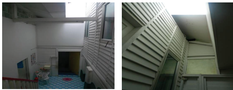
Fig.3. (a) Staircase Hallway; (b) Sky roof for natural lighting.
