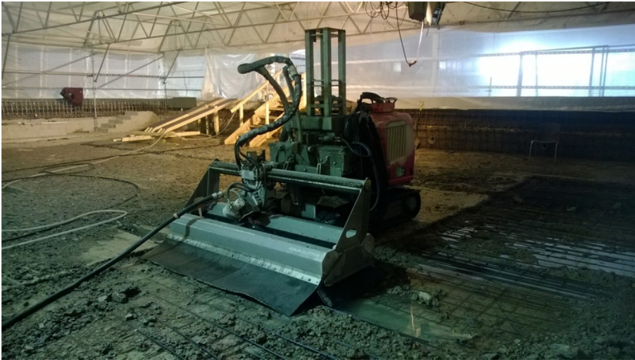
Fig. 4. The working width of the high-pressure water-jet cutter was 2 m. Concrete was removed under a temporary shield.
