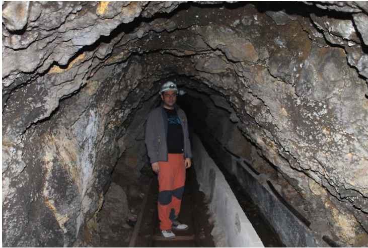
Figure 2. Inside water galleries in the Canary Islands, on the right is the channel to take out the water. At the bottom of the picture, there are the train rails for transporting material and staff.
