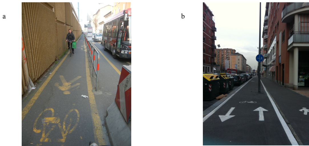
Fig. 1 – Examples of (a) insufficient width of the bike lane, or (b) presence of obstacles reducing its effective width.
