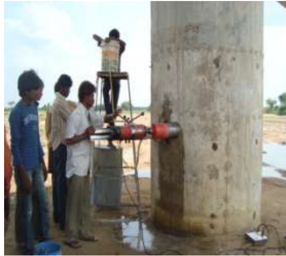
Figure 4. Extraction of Concrete core from the Bridge Pier
