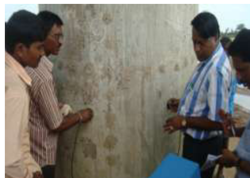
Figure 3. Testing of Bridge Pier using Ultrasonic Tester
