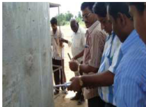
Figure 2. Testing of Bridge Pier using Rebound Hammer
