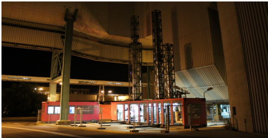
Fig. 1. The Pilot Plant at Tauron's Łaziska Power Plant, Poland.
