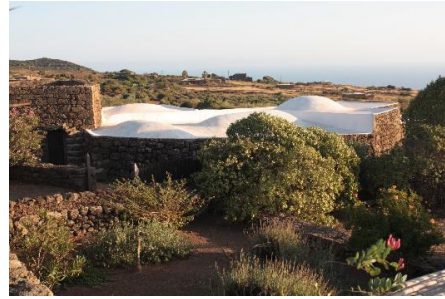
Fig. 6. Roof of Dammuso
