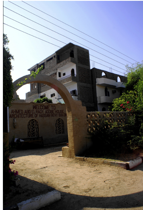
Figure 6 An example of the many uncontrolled new developments that have very modest architectural and visual qualities, which have overwhelmed New Gournia Village. These new developments, which are high-rise buildings constructed using reinforced concrete, represent a serious threat to the village authentic spirit and feeling [15].
