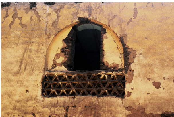
Figure 7 An example of the alterations made to the openings of one of the earthen buildings designed by Hassan Fathy in New Gournia Village [15].
