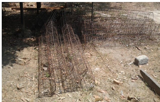
Figure 2 Reinforcement cages for making concrete pipes.
