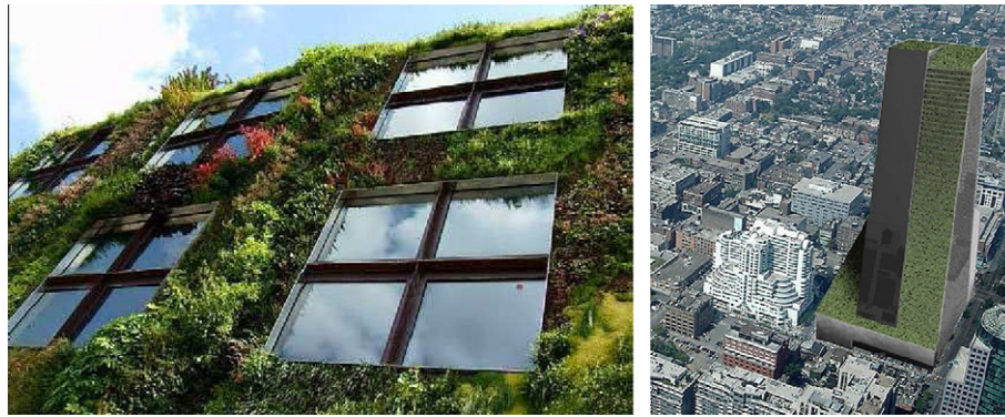
Figure 1 The cultivation of surfaces and walls in South Africa. Source: Green Building in South Africa, 2009, P. 14
