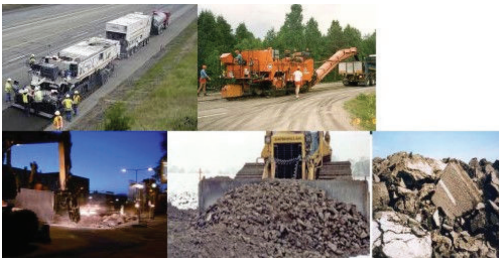
Fig. 3. Practical implementation of road demolition and recycling (the DIRECT-MAT project)
