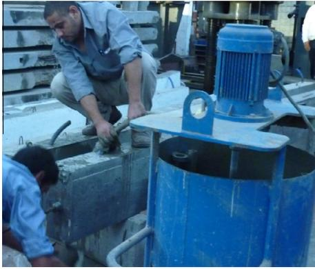
**Fig. 5** Grouting process.
