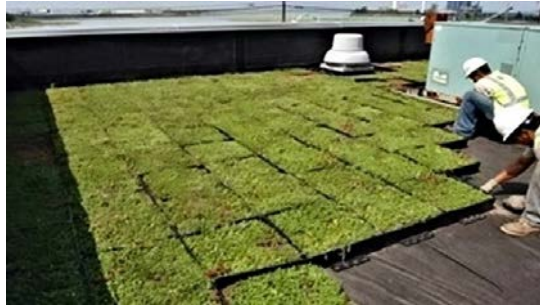
Fig. 1. Modular green roof install process.
