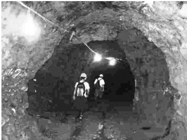
Fig. 25. Galleries in volcanic breccia unsupported.
