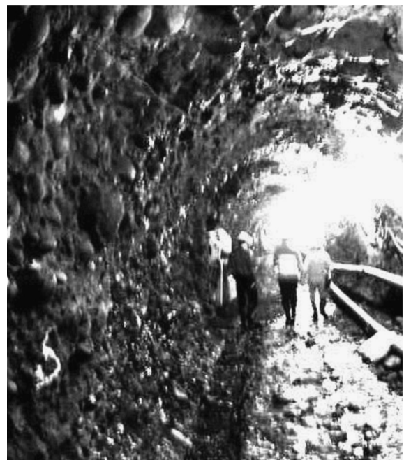
Fig. 24. Gallery in conglomerate without any support.
