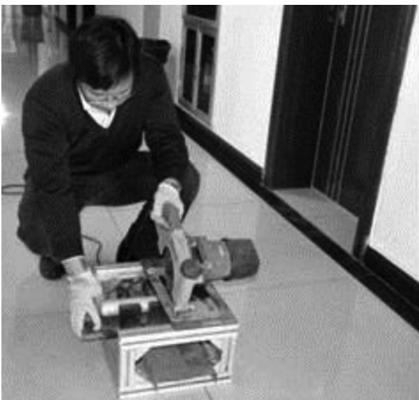
Fig. 18. Portable saw for core cutting.
