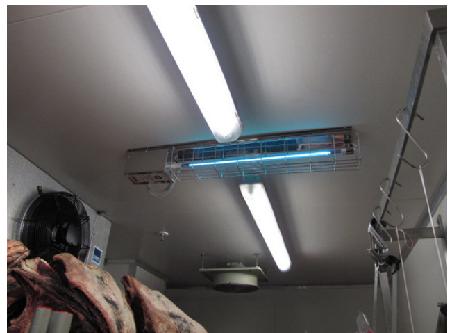
Fig. 3. Fans driving air around the room.
