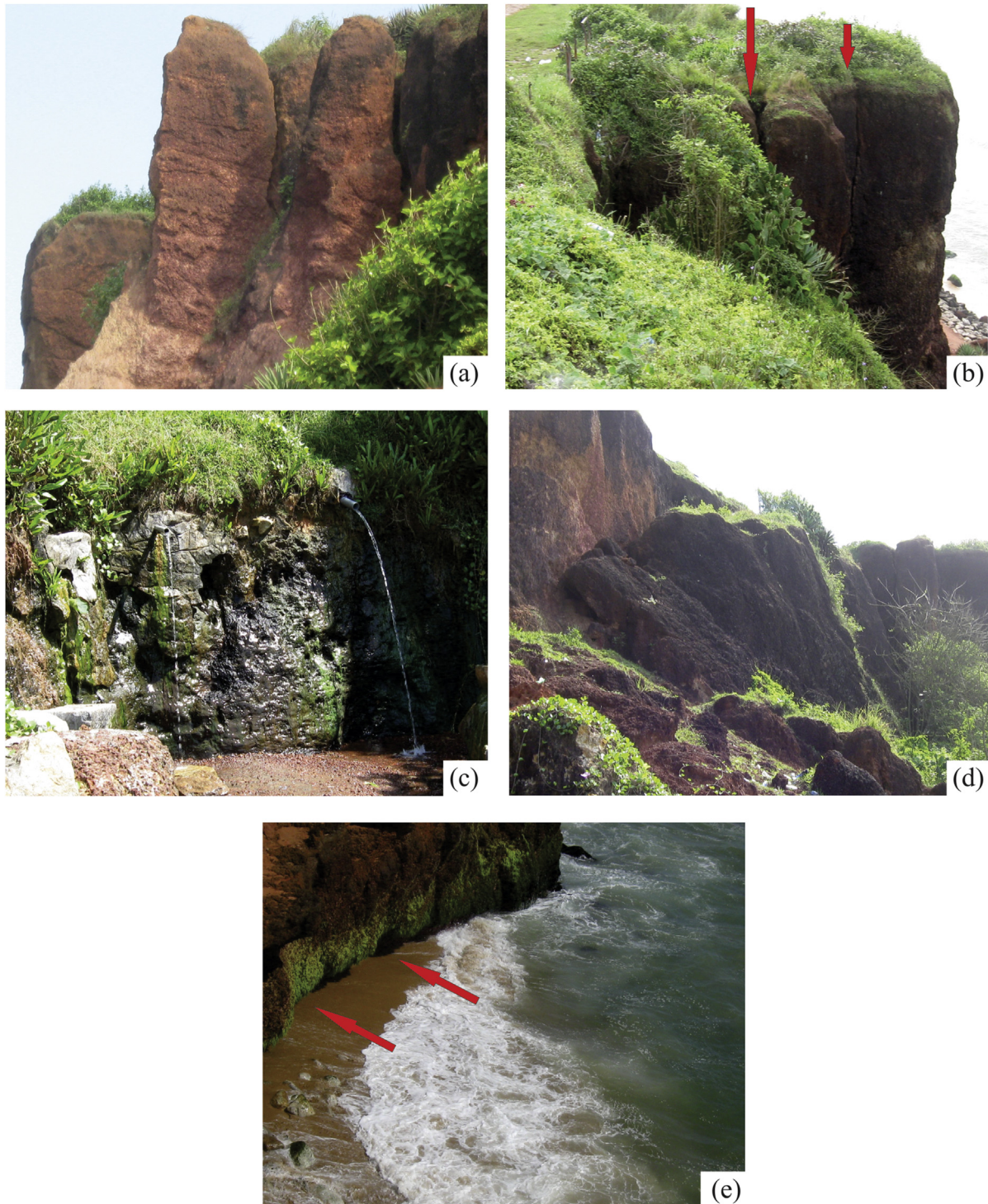
Figure 4. (a) Fall/toppling in the cliff which are the most commonest form of landslide in these cliffs. (b) Tension cracks developed in a part of the cliff. Usually these cracks are formed parallel to the cliff edge. (c) Groundwater spouting as springs at the contact of sandstone and carbonaceous clay in the cliff. A spring line exists all along this litho-contact. (d) Slippage which is mainly initiated by wave erosion and fail along planes which will be usually concave in shape. (e) Sea notches formed by wave action. Less resistant material will be eroded fast than the most resistant ones.
