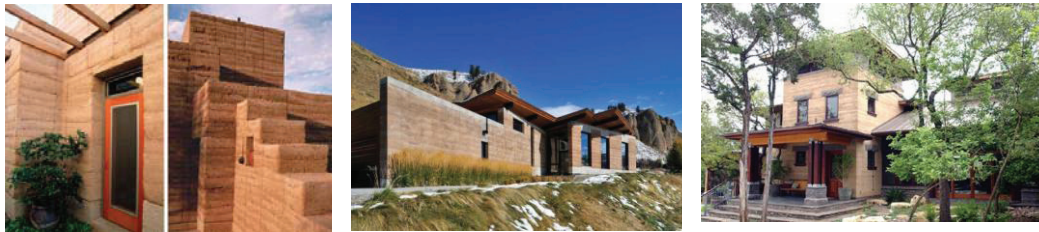
Figure 4: Rammed Earth Home by Paul Weiner [13]
