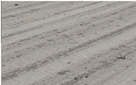
Fig. 7. Compacted fine seal.
