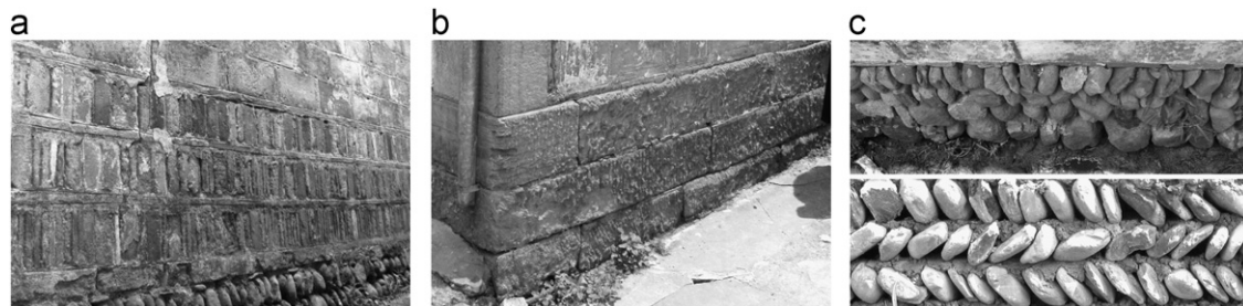
Figure 2 Common wall materials in Hui-style vernacular dwellings: (a) clay brick, (b) natural granite stone, and (c) pebble. (For interpretation of the references to color in this figure legend, the reader is referred to the web version of this article.)
