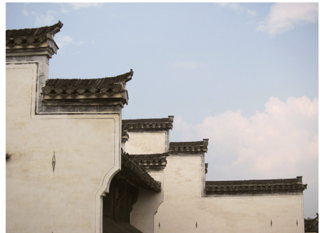
Figure 7 Horsehead walls as a distinct architectural feature of the Hui-style vernacular dwellings.
