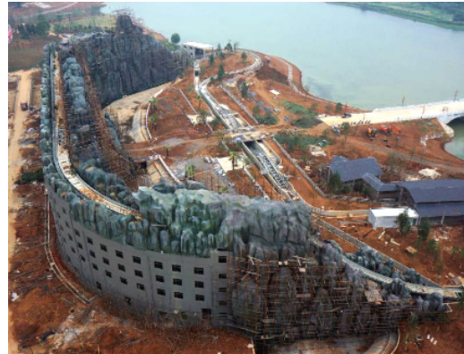
Fig.3: right facade image of the landscape by UAV
