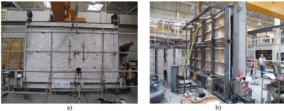
Fig. 4. General view of the experimental test setup a) Front view b) Lateral view.
