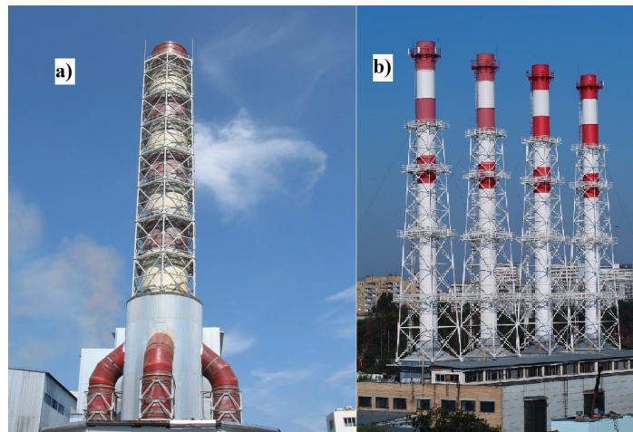
Fig. 1. Fiberglass gas exhaust ducts: (a) with the diameter of 5,0 m at the plant named after A.K. Serov, the city of Serov; (b) with the diameter of 3,25 m at the regional heating station Birulevo, Moscow.
