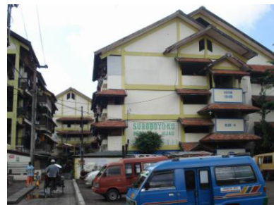
Fig. 4 Sombo housing in Surabaya, Indonesia. Source : field survey, 2012
