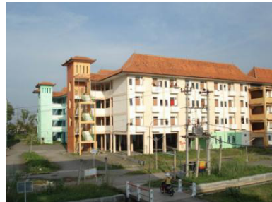
Fig. 2 Kaligawe housing in Semarang, Indonesia. Source : field survey, 2012
