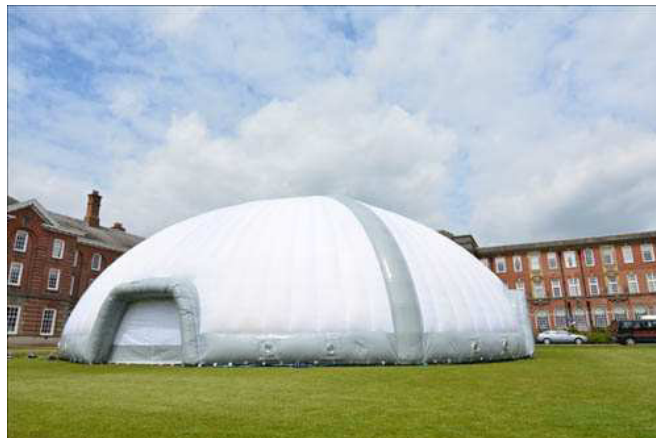
Fig. 4: 20 Metre Span Dome Structure (Image by Ingenious)
