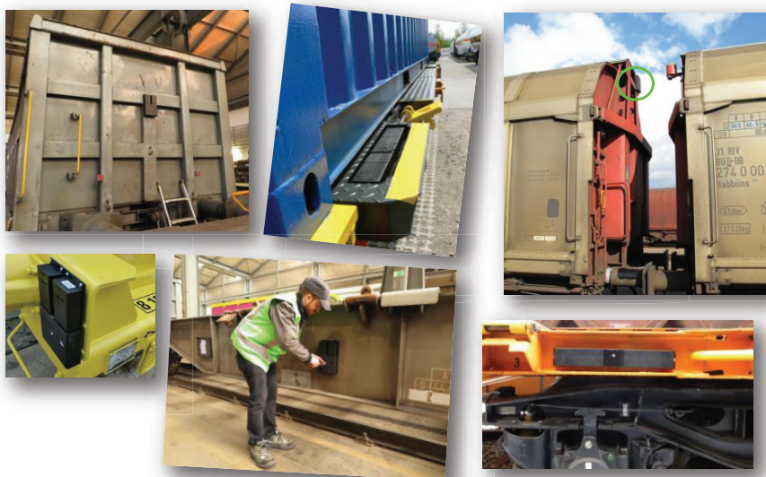
Fig. 4. aJour Telematics installation examples (source: Eureka).
