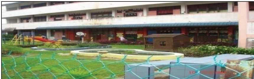
Figure 2.2 Front view of the renovated public preschool classroom
