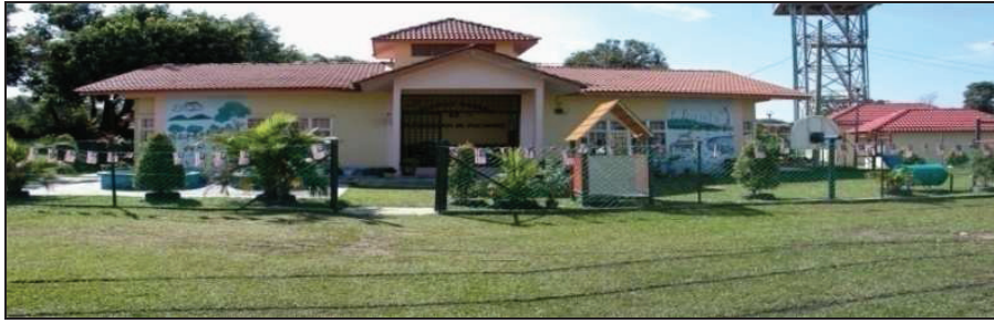
Figure 1.2 Front view of new preschool building (annex building) with two classrooms
