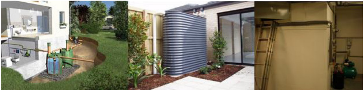
Fig. 2. Underground rainwater tank, over ground rainwater storage reservoir, and storage reservoir as a part of basement disposition [5, 6]
