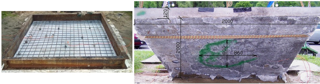
Figure 2 Casting of the reinforced concrete slab and cracks at the lower surface of the failed reinforced concrete slab after its lifting up.
