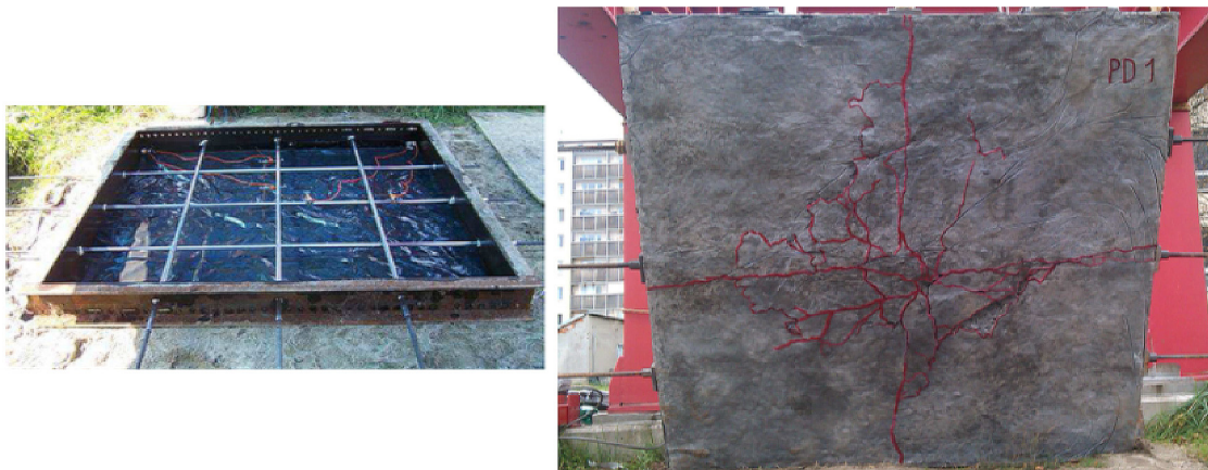
Figure 3 Casting of the post-tensioned concrete slab and cracks at the lower surface of the post-tensioned concrete slab after its lifting up.
