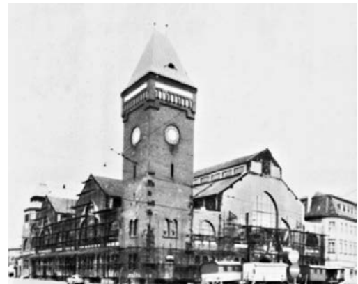
Figure 7. View of the front façade during repair works in 1980-83, [14].
