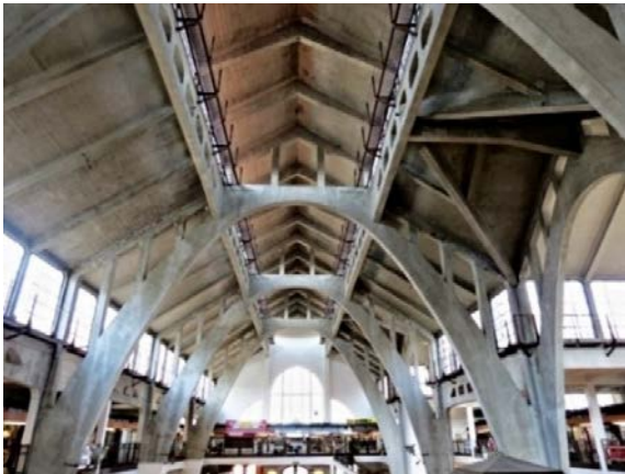
Figure 2. View of the main structural arches.
