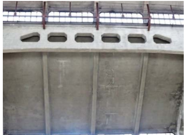
Figure 3. View of the castellated stiffening beams.
