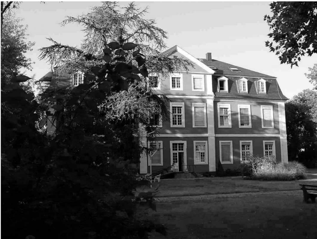
Fig. 1: The 'Schloss'. Two inpatient wards of the Clinic for adults are accommodated here before the new hospital building is completed. In the basement, the outpatient section for severely handicapped persons and the outpatient EEG labs are located.
