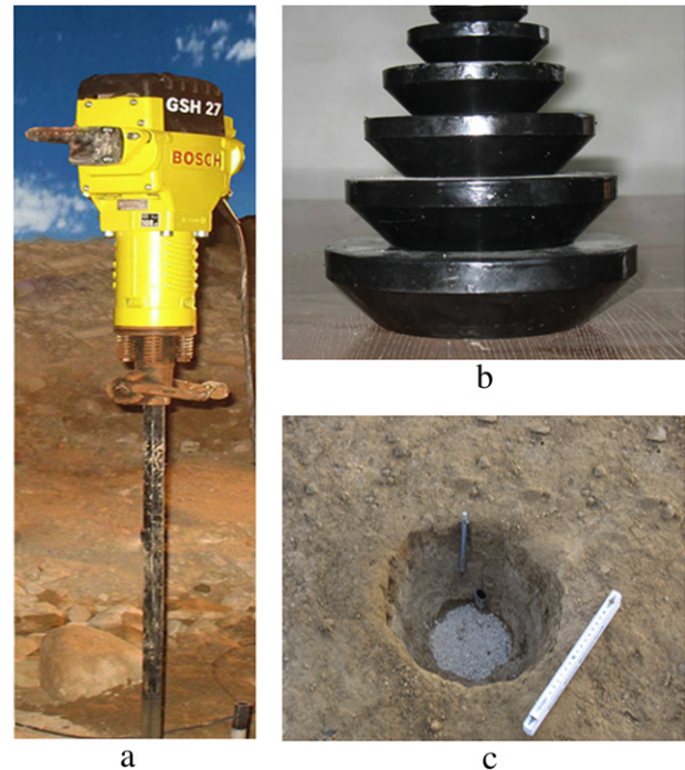
Figure 1: Illustrations of (a) electric rammer, (b) special tampers by 45 degree bezel, and (c) a typical of RAPs after loading.
