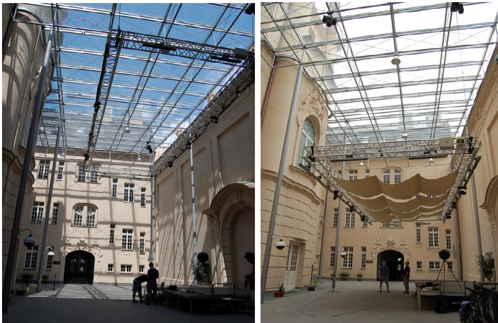
Fig. 1. Interior of the atrium of Slovak philharmonic in Bratislava with and without absorptive material placed over the stage
