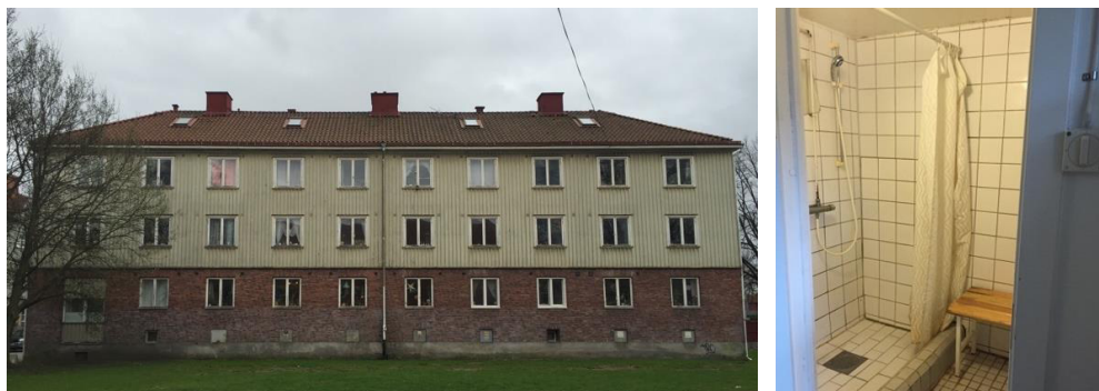
Fig. 4. Case study building 1 is a Landshövdingehus on Banérsgatan 6. Left: façade with brick on ground floor and wooden weather board on the upper two floors. Right: common shower in basement.
