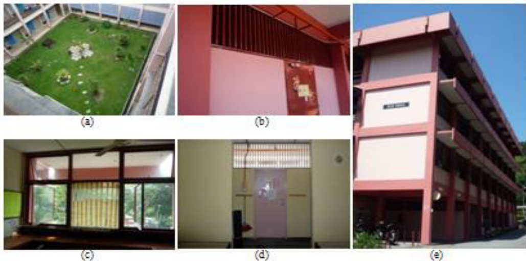
Fig.. 2. (a) Square internal courtyard; (b) Fixed transom on top of the entrance door and internal walls; (c) Types of windows – centre pivot and awning; (d) Wall opening in the room; (e) Large horizontal overhangs along the windows
